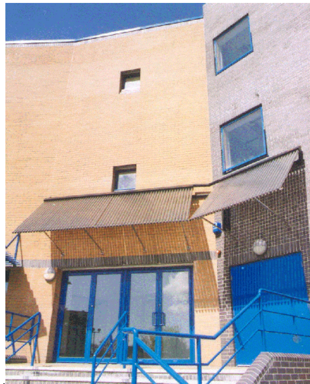
Figure 6: The flexibility and low wind resistance of Thermomax tubes offer unique designs. They are used as awning in the above installation.
