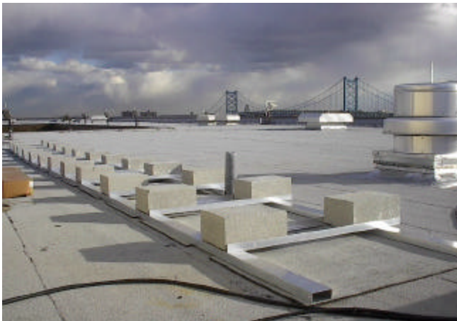
Figure 9. Thermomax collectors will be anchored on four Ballast blocks.
