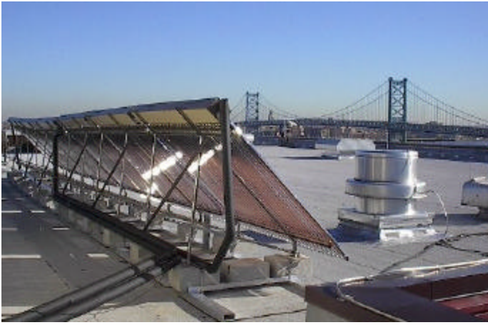
Figure 1. Photograph of the solar array on the southwest riser of the building recirculation loop on the Mid Atlantic Social Security Center, Philadelphia PA. The other array on the northeast riser is identical in size and orientation.
